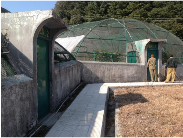
Enclosures outside view
