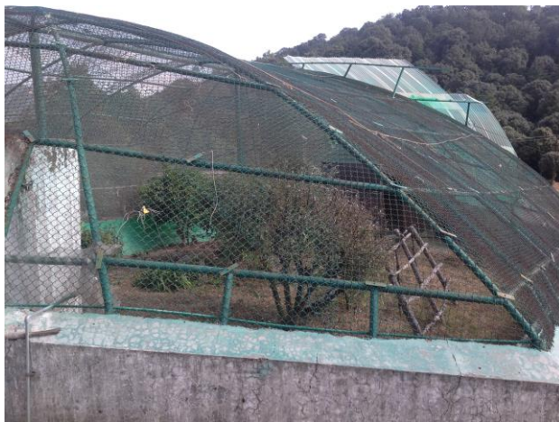
Enclosure as seen from outside
